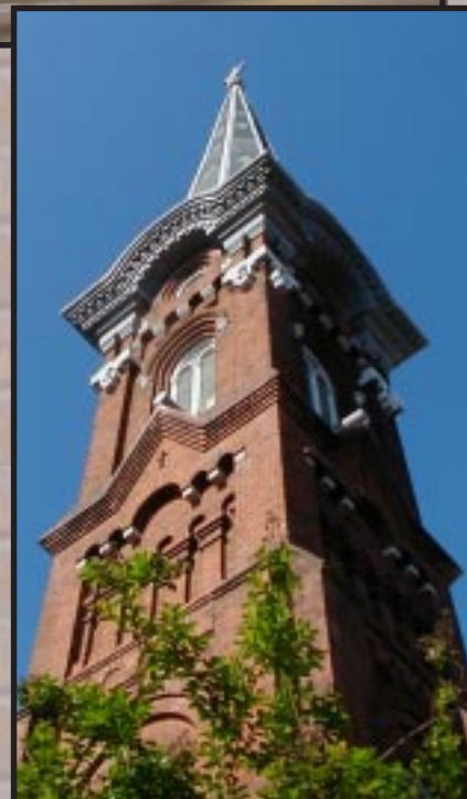
This marvelous structure is comprised of 1,265,870 bricks that were fired on the construction site. Holy Trinity's 170-foot tall tower (right) can be seen from many places in the town of Vicksburg.
