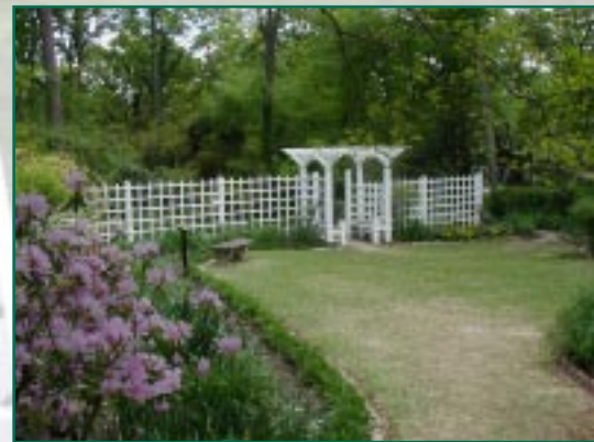
The original wooden trellis and arbors were replaced with new ones made from structural steel.
