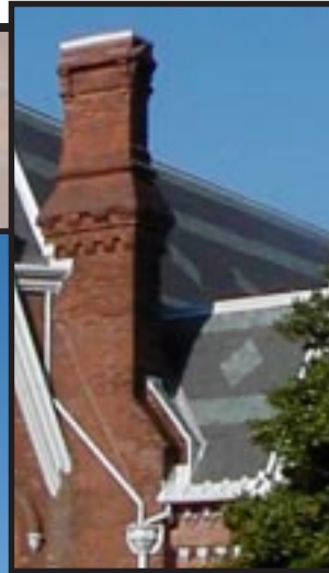
The roof was reslated in 1997 with slate imported from Belgium, replacing the original Belgium slate that had lasted for 117 years.
