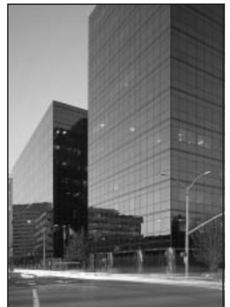
City Centre: A new parking garage is being built for City Centre to accommodate new and expanding tenants.
