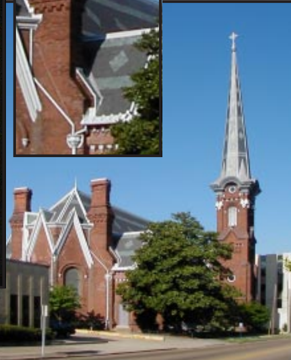
The roof was reslated in 1997 with slate imported from Belgium, replacing the original Belgium slate that had lasted for 117 years.
